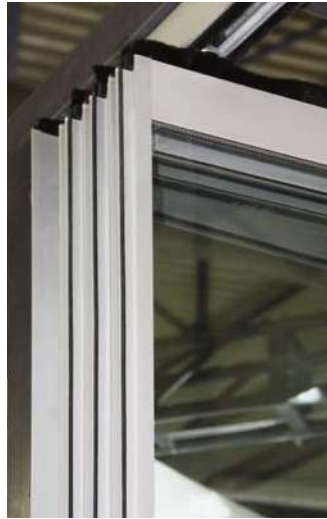
High resistance female & male vertical profiles for the maximum weather proofing between framed panels.
